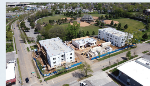
Aerial view of Caswell Manor under construction.
